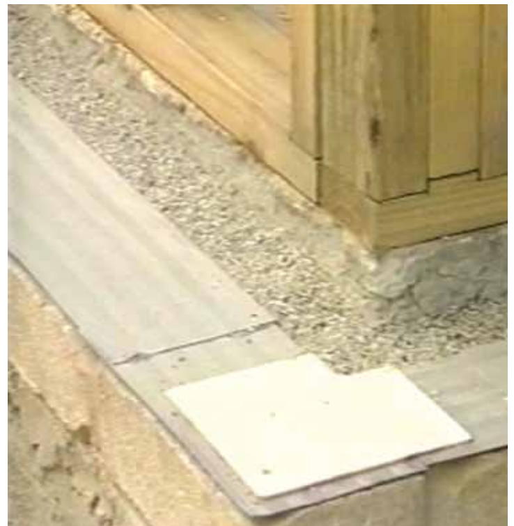
Under floor graded stone fill treatment (minimum compacted depth 75mm). Alternatively the underfloor graded stone can be omitted and the penetrations through the slab protected by an approved system
